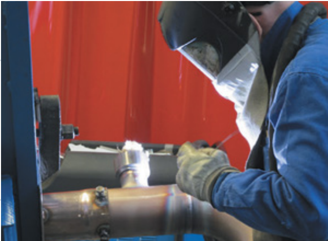
Welding CuNi piping spools
