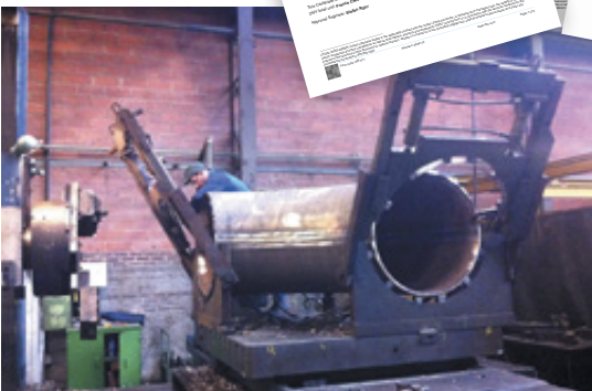
36" CuNi welded elbows
