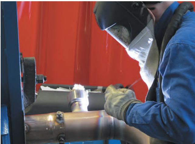
Welding CuNi piping spools
