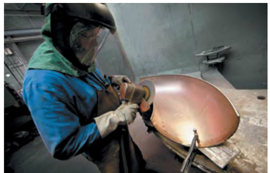
End preparation before welding half shell CuNi elbows
